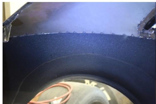
Panel & Wedge Tacked into Place - Inside
