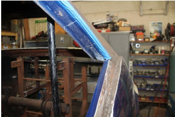
Front View Drip Edge Moved & Welded
